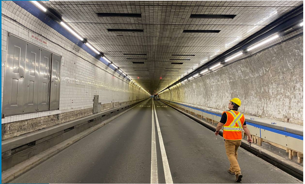
G&G engineer inspecting the installation. Notice the contrast between the newly installed PRX fixtures and the old fluorescents in the background.
